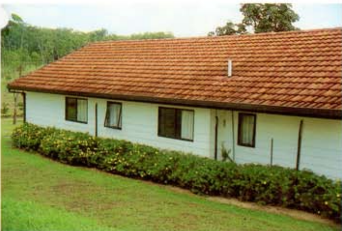
Supertex Woodgrain Planks Used For External Cladding In This Residential House, Kajang Country Heights.
