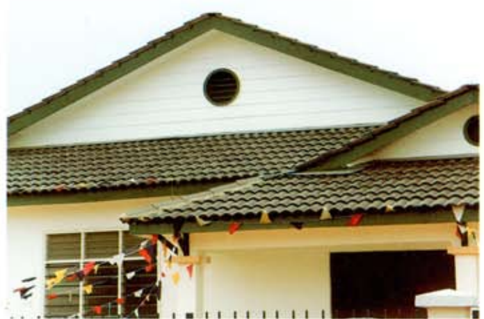
Supertex Woodgrain Planks Used For Gable Ends In A Residential House, Permas Jaya, Johor.
